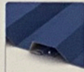
Detail of HR-16 Panel Interlock
